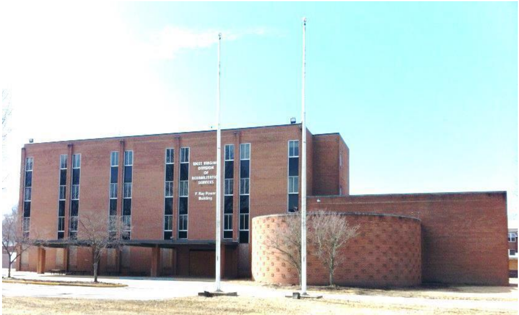
Figure 3. The F. Ray Power Building, located at the new WVSU Research Station site
